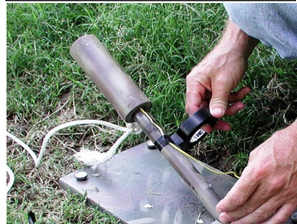
Figure 5c. Taping the electric match leg wires to the launch rod to keep it in place.
