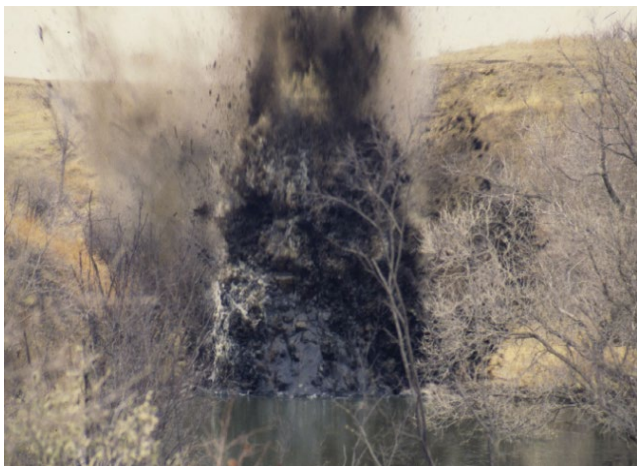
Figure 3a. Blowing up a beaver dam with explosives. Blasts are intentionally directed to minimize potential damage to nearby structures.
