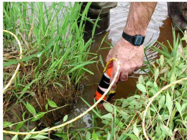
Figure 1c. Placing an explosive charge attached to detonating cord.
